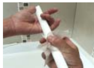
Take the appropriate 1m profile and fit it to the long profile behind taps - Mark to size - Cut and fit "dry" - Repeat with remaining profile
