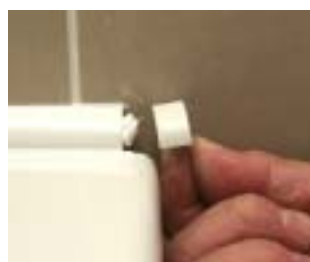
Change to fine nozzle - Seal in top and bottom of profile with silicon - Fit End Caps - Use Fugi 2 to remove excess silicone - Leave to Set ( 4 Hours )
