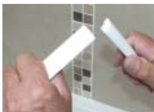
Take the appropriate 1m profile and fit it to the long profile behind taps - Mark to size - Cut and fit "dry" - Repeat with remaining profile
