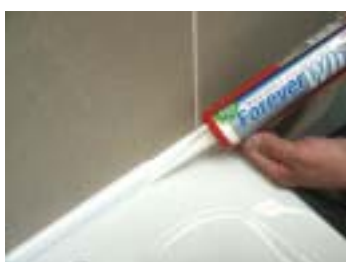
Change to fine nozzle - Seal in top and bottom of profile with silicon - Fit End Caps - Use Fugi 2 to remove excess silicone - Leave to Set ( 4 Hours )
