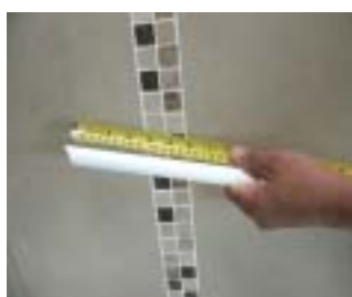
Measure length of bath and transfer measurement to 2m profile - Mark and cut to length by scoring and snapping profile - lay on bath "dry"
