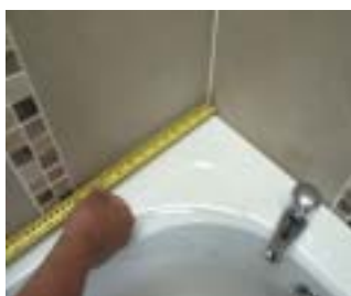
Measure length of bath and transfer measurement to 2m profile - Mark and cut to length by scoring and snapping profile - lay on bath "dry"
