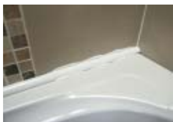
Clean Profile - Fit the long length 1st - Add generous silicone with large nozzle - Fit profile and remove excess with Fugi 2 or finger - Now fit end pieces
