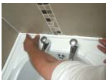
Change to fine nozzle - Seal in top and bottom of profile with silicon - Fit End Caps - Use Fugi 2 to remove excess silicone - Leave to Set ( 4 Hours )
